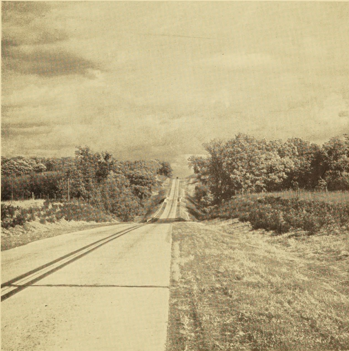
NATIVE PLANTING ON SLOPES INACCESSIBLE TO MECHANICAL MOWERS ON ROAD NEAR ELDORA, IOWA
